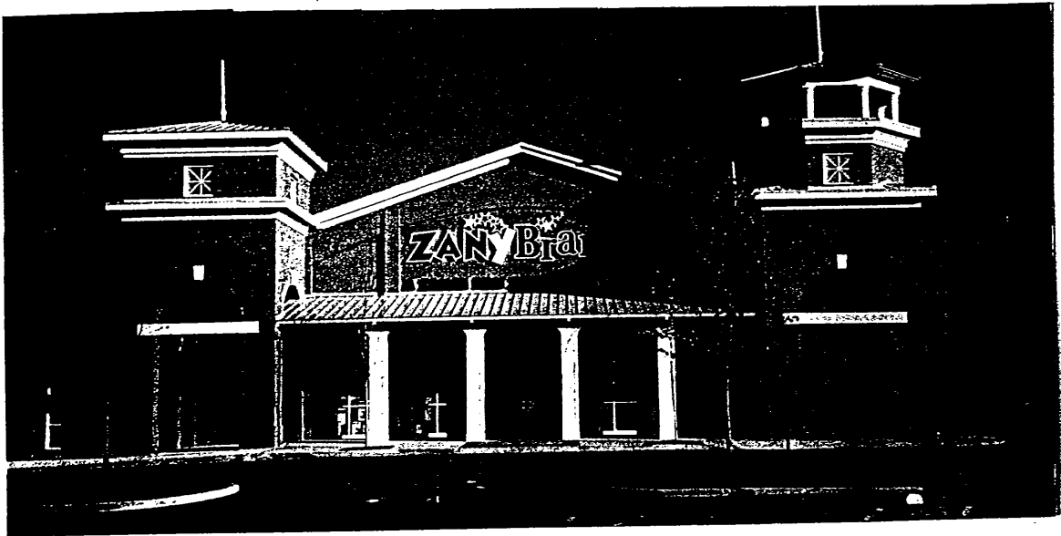
Highly visible entryway with weather protection features
